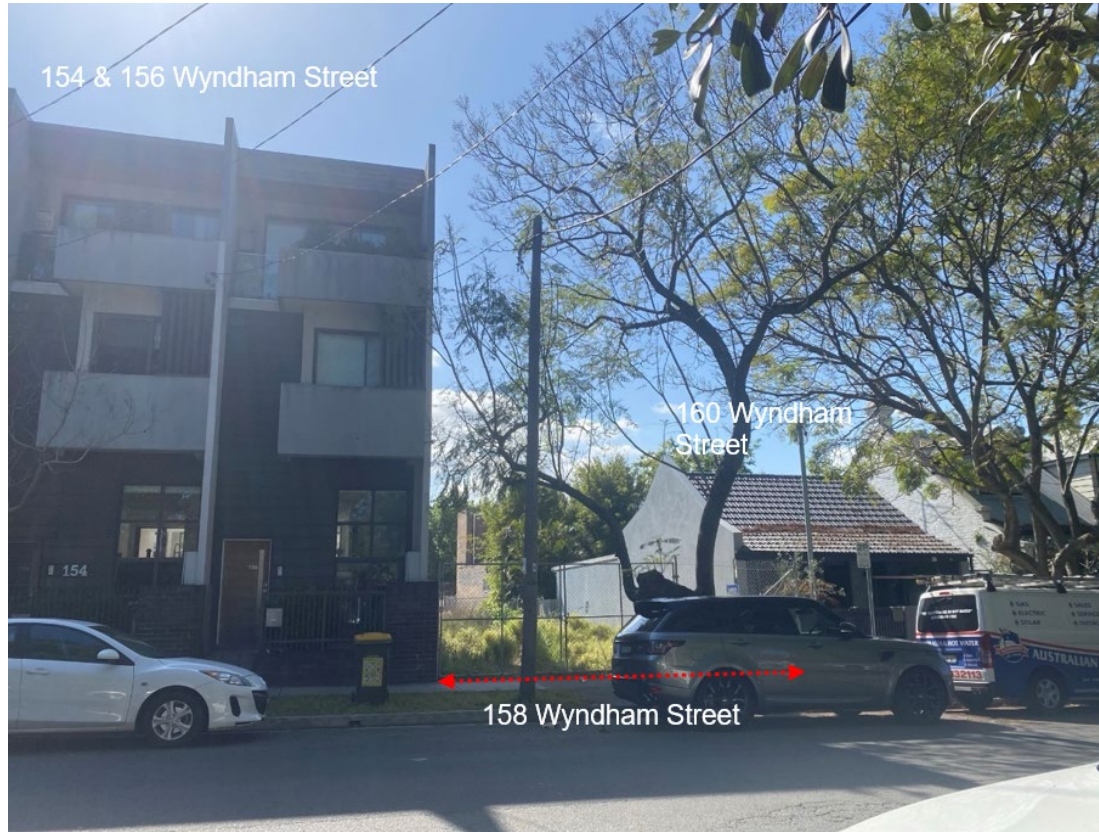
site viewed from Wyndham Street
